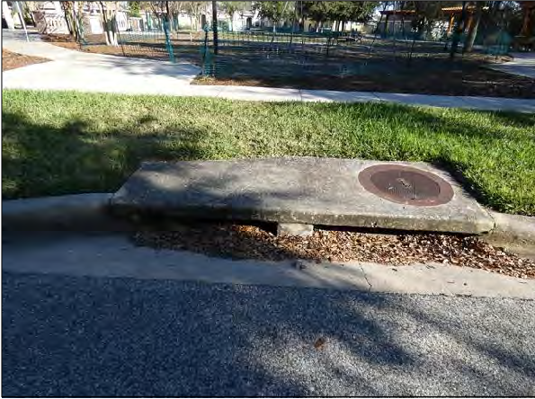
Stormwater Drainage Curb Inlet
